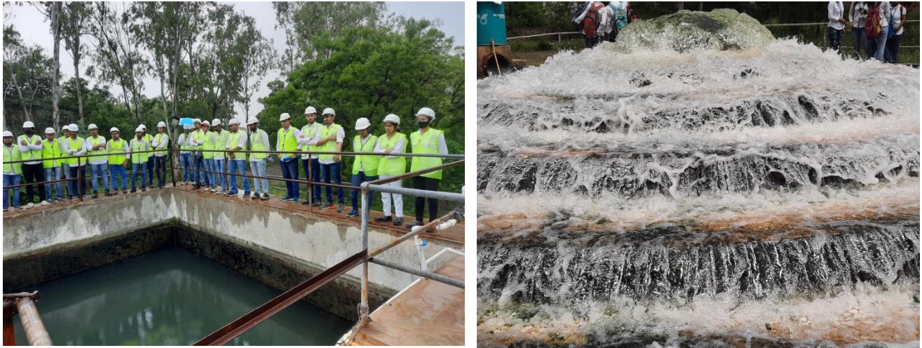
Figure 6: Images of Pharola WTP
